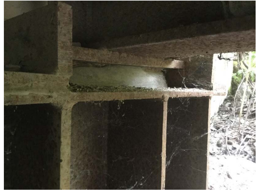
Upstream right bank bearing, 60mm from stream side cap face
