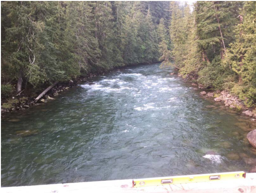
Looking upstream from deck
