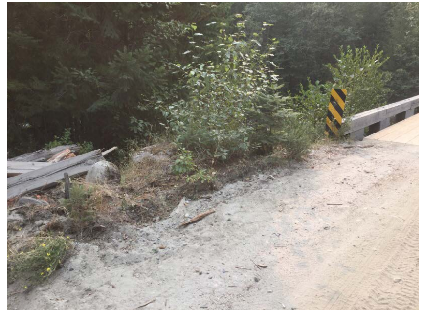
Downstream left approach fender
