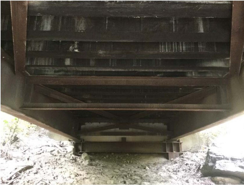
Jump span superstructure
