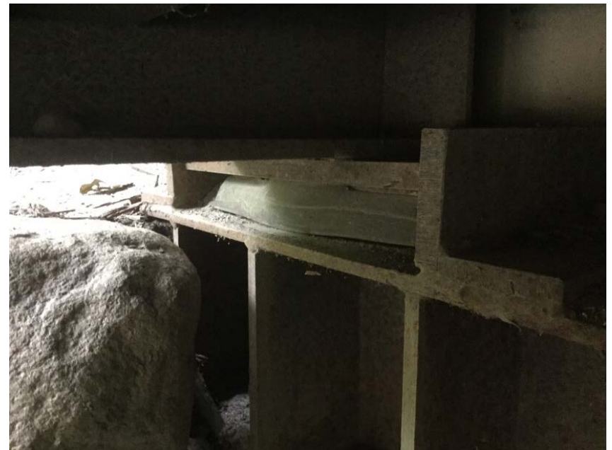
Downstream right bank bearing 30mm from stream side cap face
