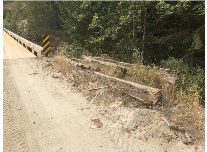
Upstream left approach fender
