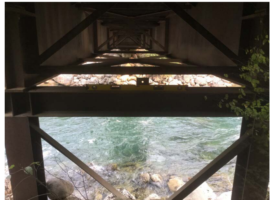
Main span Superstructure and bent
