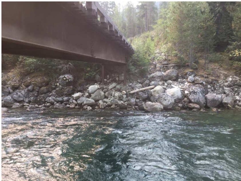
Right Bank Abutment when facing downstream
