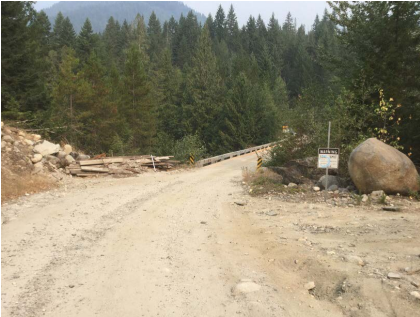
Approach from Right Bank when facing downstream
