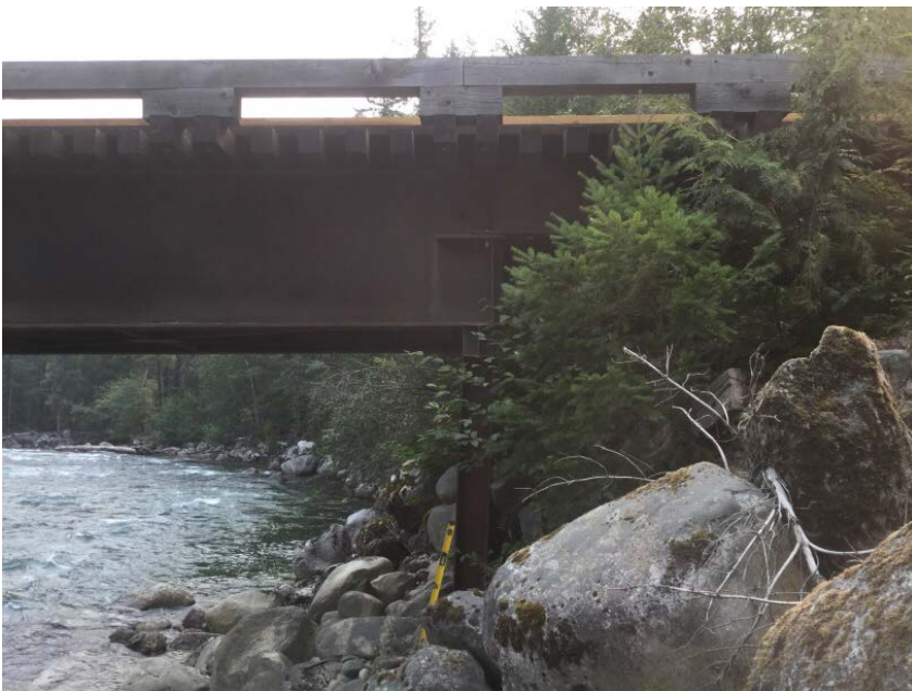
Jump span seat and support not vertical
