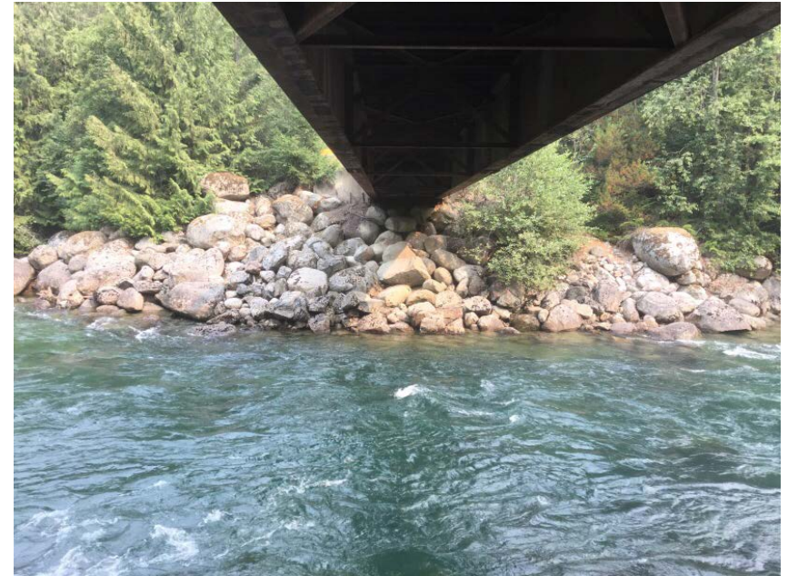
Left Bank Abutment when facing downstream
