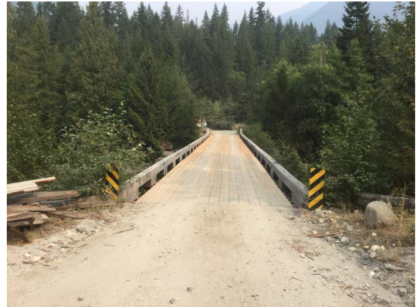
Approach from Right Bank when facing downstream
